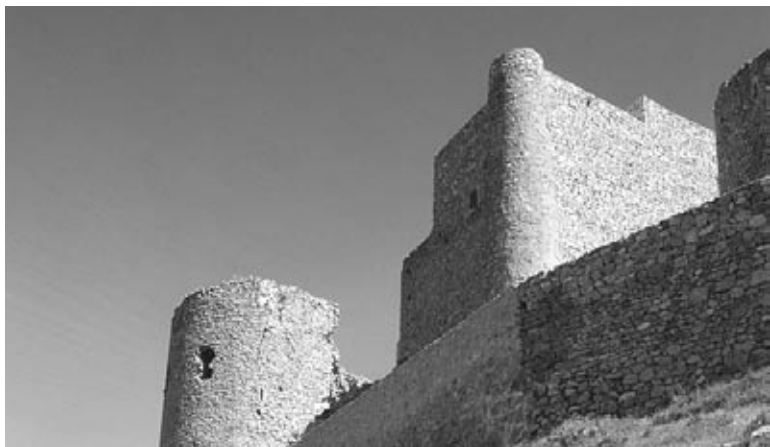
Curtain wall and turret of the outer bailey. The keep is also visible.
